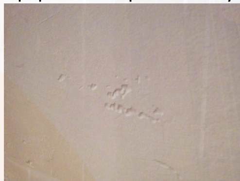
Oil / grease / moisture trapped below paint - Blistering
